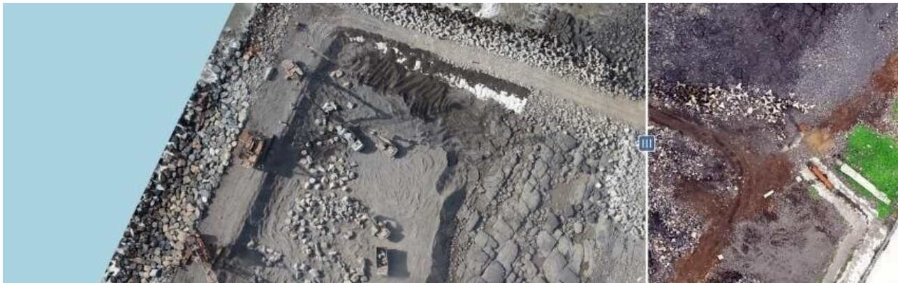
Georeferenced drone orthomosaic of the ship recycling yard
